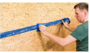
2. Taping of panel joints Centre TESCON RAPIC on the joint, roll it out and stick the panel joint gradually.
